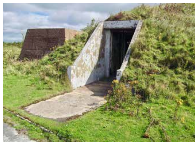
The Variable Elevation Beam building located below one of the receiver masts. The concrete base of the mast is seen on the left. Photo Adrian Armishaw
